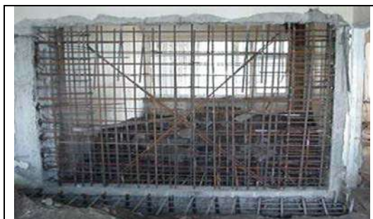
(Fig – 87 Additional Shear Wall)
