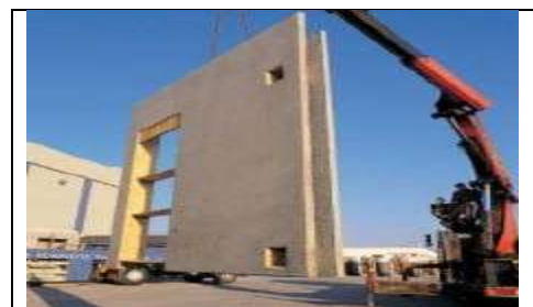
(Fig – 93 Precast Flat Panel System)
